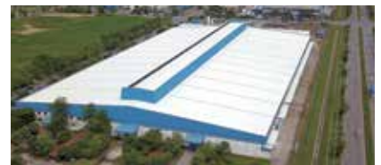
Fujitsu General (Thailand) Co., Ltd. (Thailand) FACTORY-2
